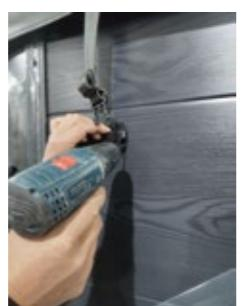
Step 4 - Use a screwdriver to finish screwing in the 3 screws. (Repeat this process for the other 3 corners.)
